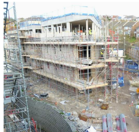
East block under construction
